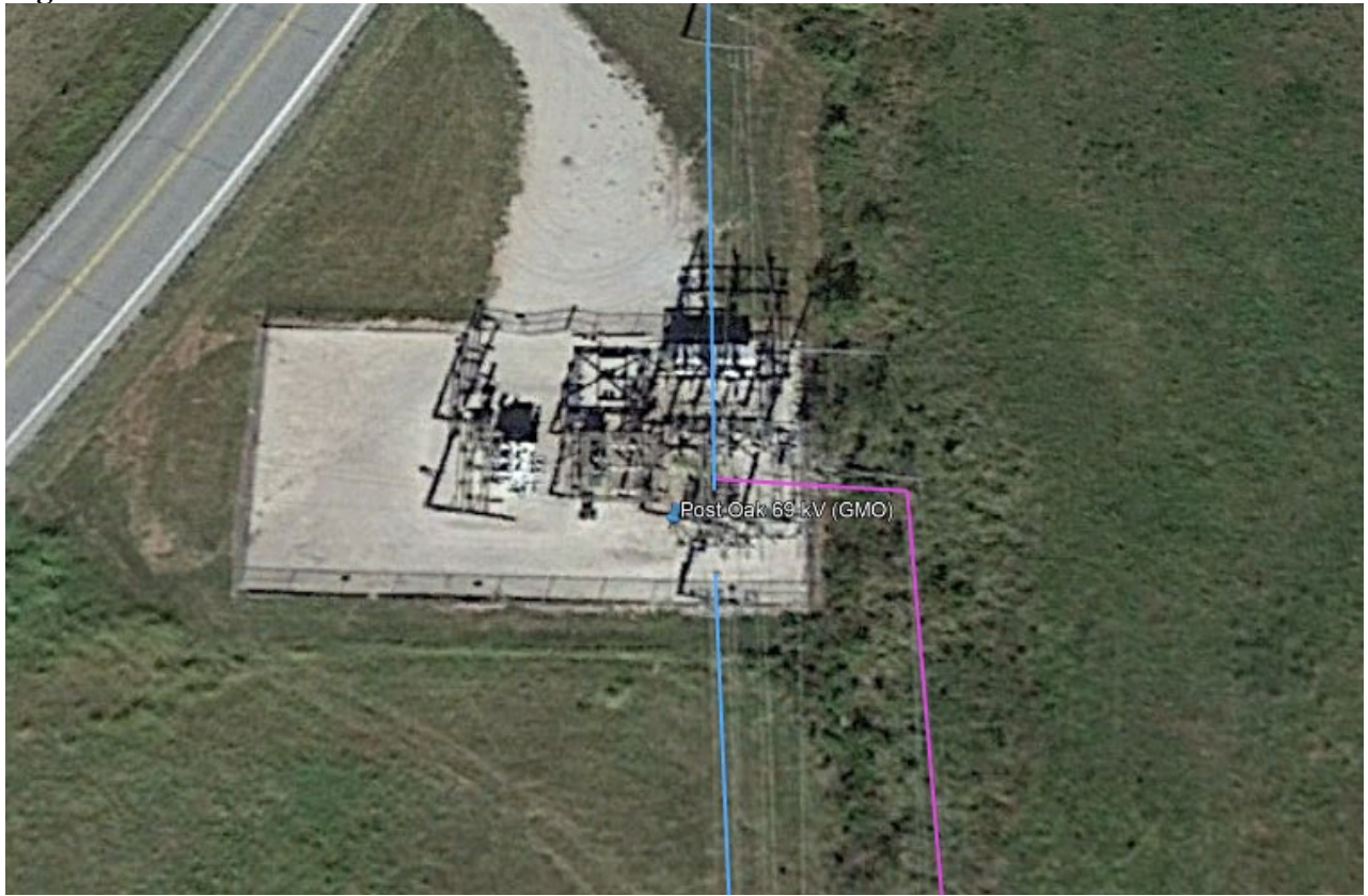
Figure 14 – Post Oak – 69kV Transformer
