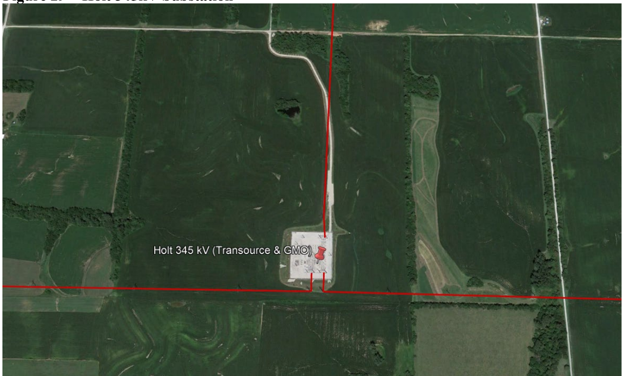
Figure 29 – Holt 345kV Substation
